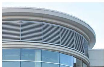
Although these louvers were installed only for aesthetic purposes, the Airolite Louver Type 609 is designed for applications that require intake and exhaust ventilation with moderate protection against water penetration.
